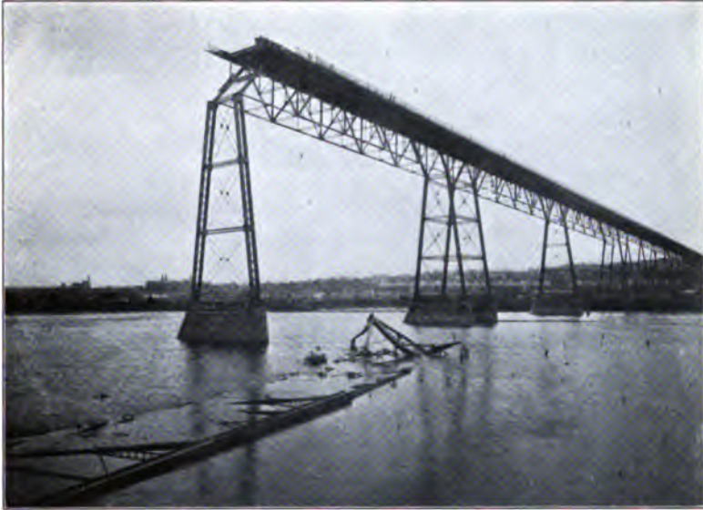
FIG. 1.—SMITH AVE. VIADUCT. VIEW LOOKING NORTHWEST. WRECKED BY STORM OF AUGUST 20TH, 1904.
